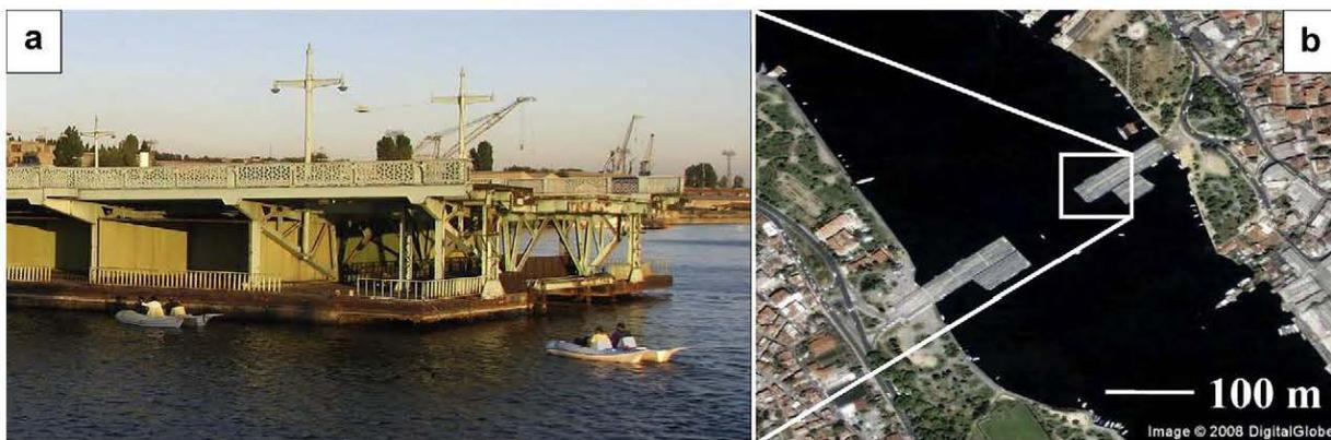
**Fig. 7 – Side view from the north (photo a) and aerial view (photo b; ©Google Earth) of the Valide Sultan/Old Galata Bridge after 2000 with the two center sections removed.**
