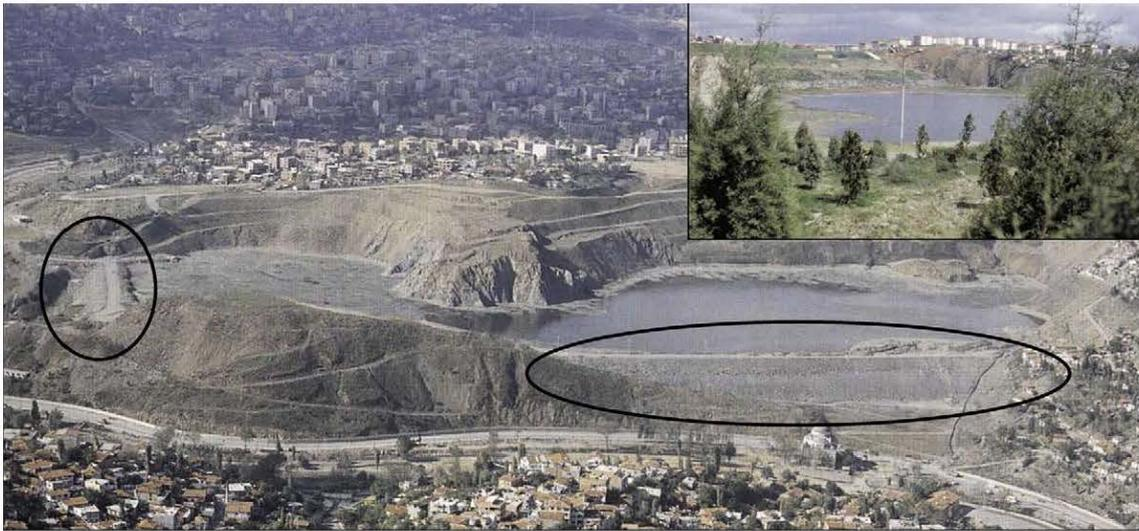
**Fig. 6 – The Kucukkoy dams in 1998 during sludge filling (dams are circled), and post-dredging (inset) when sludge was covered with soil to create a recreational area (© ISKI).**
