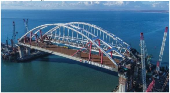
The roadway arch of the Crimean Bridge has been raised onto its fairway supports and securely attached at the planned height of 35 meters above the water. Shipping on the Kerch-Yenikale Canal resumed at noon – 18 hours ahead of schedule.
