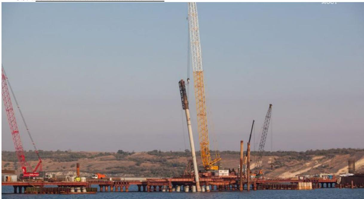
Construction workers have finished sinking piles on the road section of the bridge across the Kerch Strait. The last tubular pile was driven into the ground at support No. 256 in the waters between the fairway and the Kerch shore. The road's foundations consist of over 3,000 piles.
