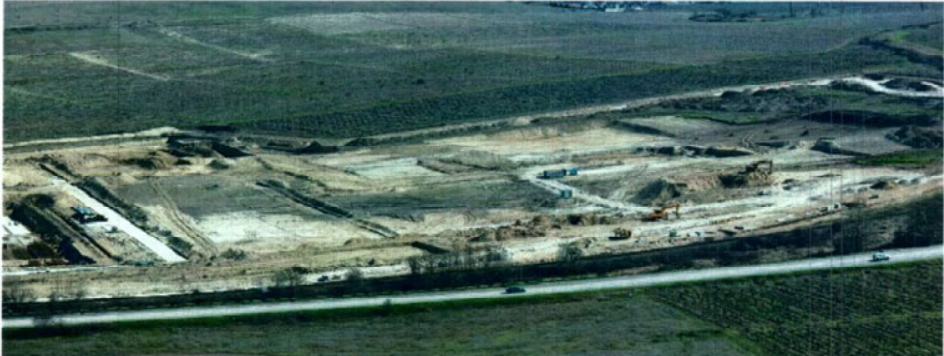
Start of construction CCP-TPS (Simferopol and Sevastopol)
