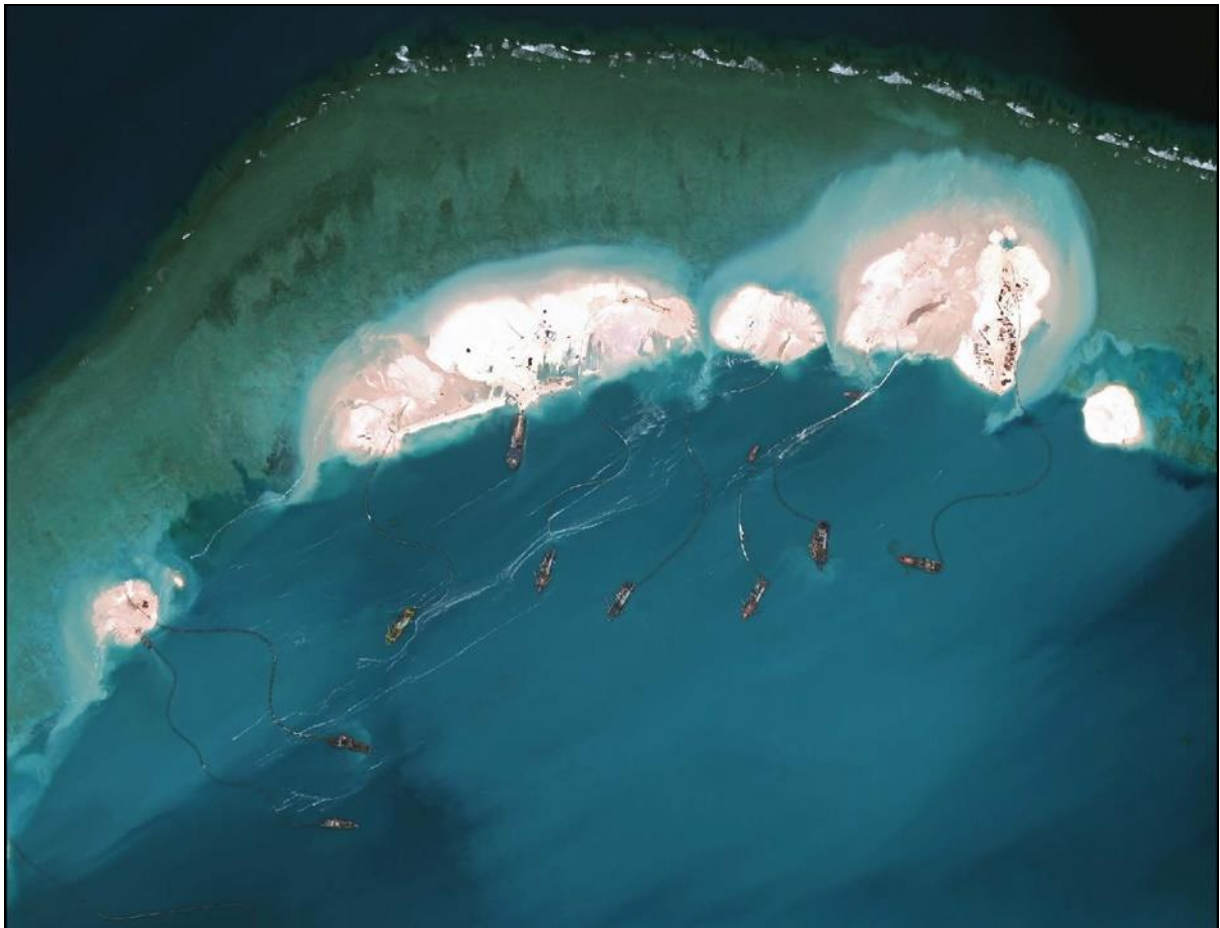
Figure 17: Dredgers at work at Mischief Reef (Annex 792)
