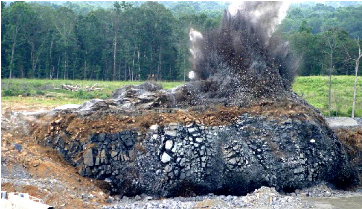
Figure 6. Photograph of Blast 2904 soon after initiation clearly showing oversize blocks in the free face and stemming region.
