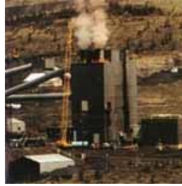
The coal preparation plant.
