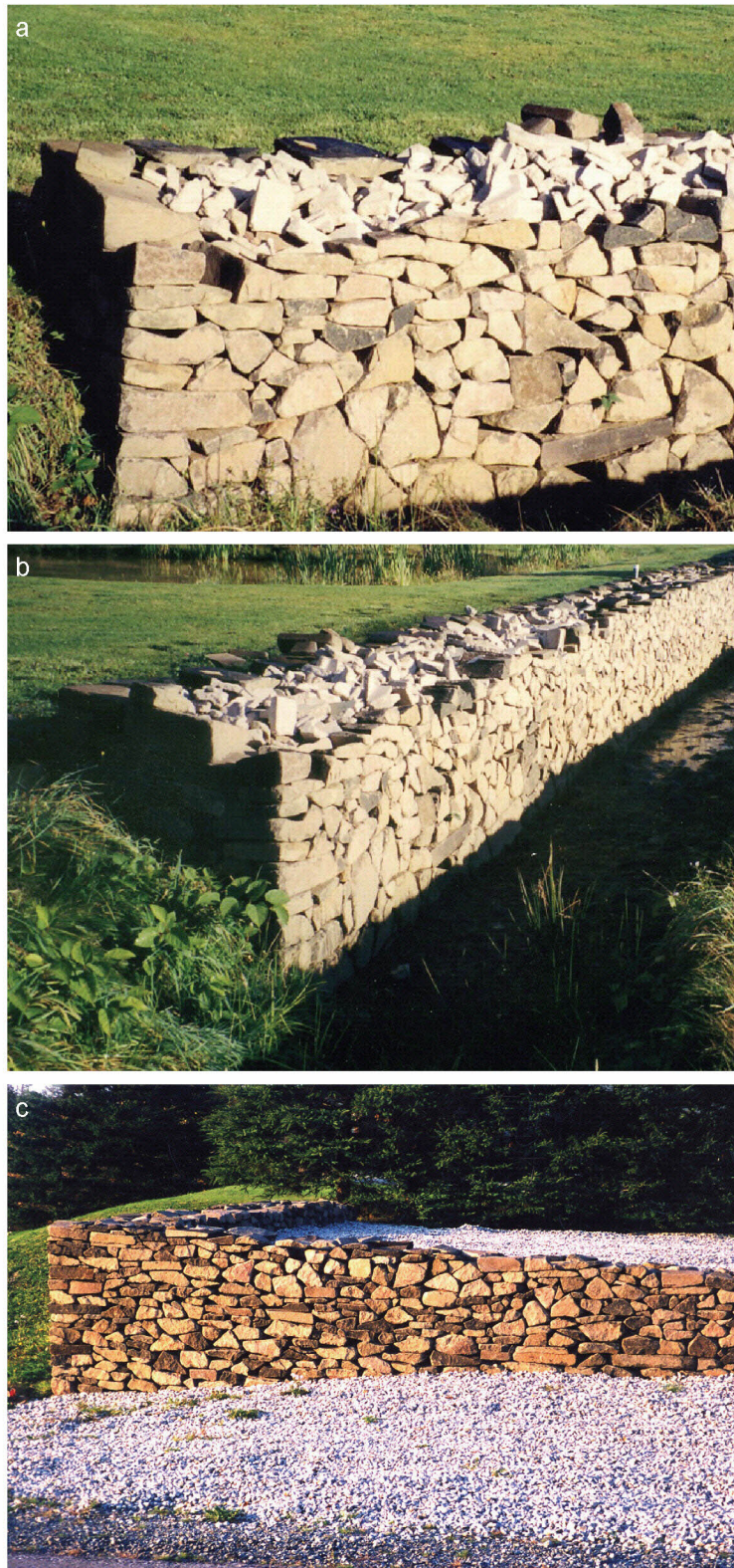
Figure 8a, b, c. Examples of columnar-jointed basalt stone walls. Figures 8a and b show a free standing dry-stone fence (in progress) with two finished faces and a centre filled with rubble. Note the rectangular shape of the corner stone and flat pieces being placed for the top course. Figure 8c is a retaining wall supporting a raised driveway. Notice the variety of stone shapes and colours in this wall as well as the rectangular-shaped corner blocks.
