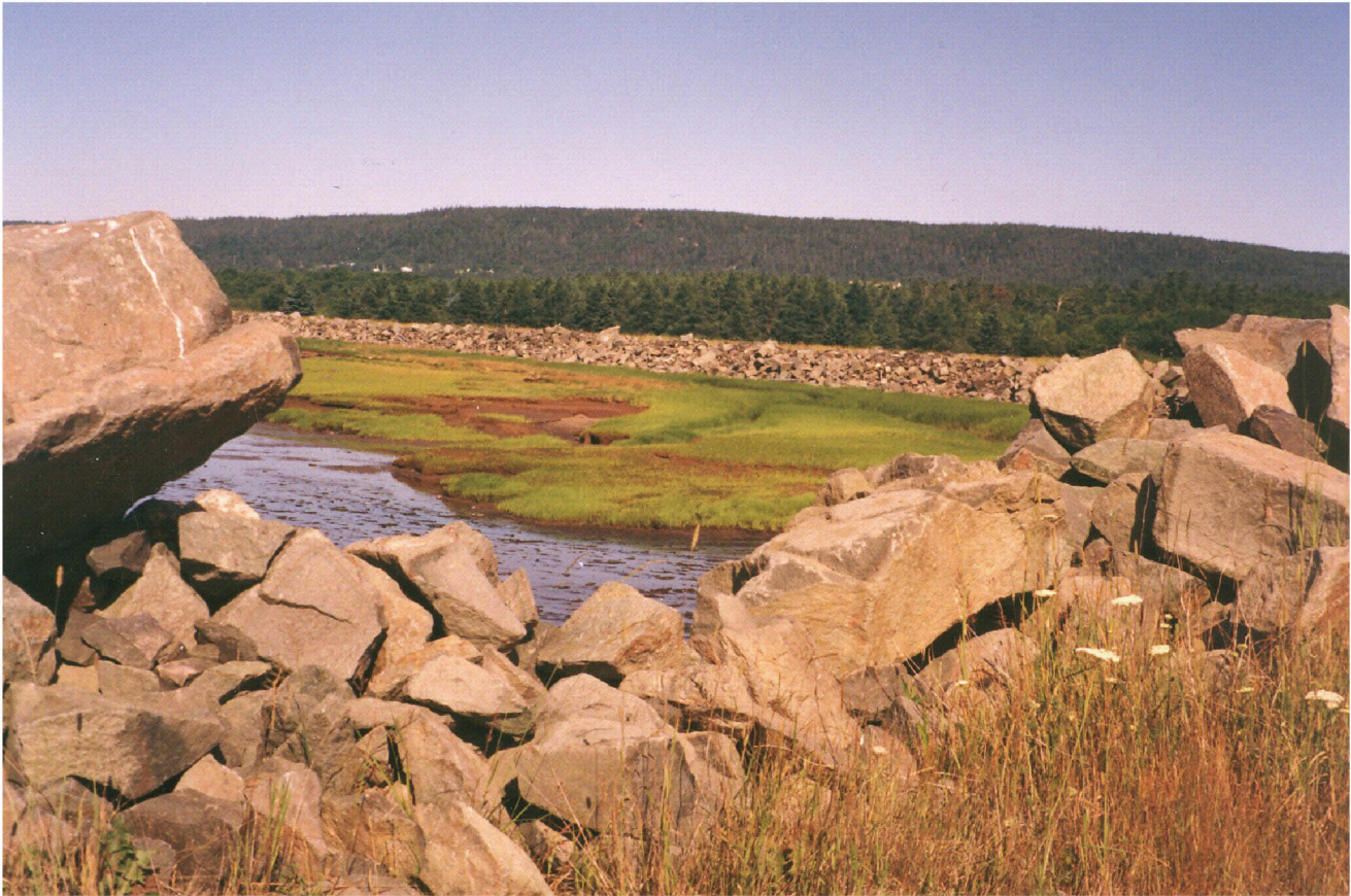
Figure 10. Basalt armourstone used to protect a dyke from erosion at the head of St. Marys Bay near Roxville, Digby County.
