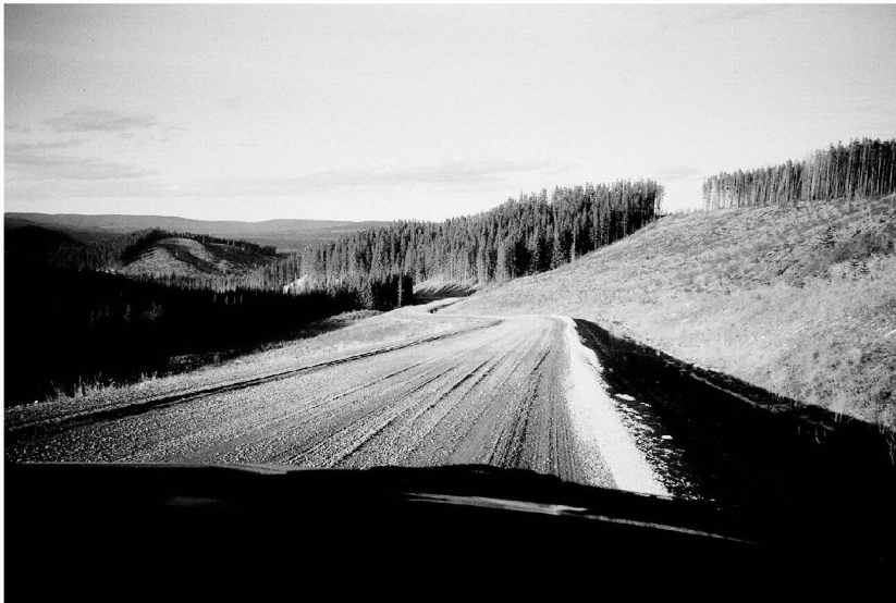
Photo No. 2: Mainline Road (5 November 2002)
