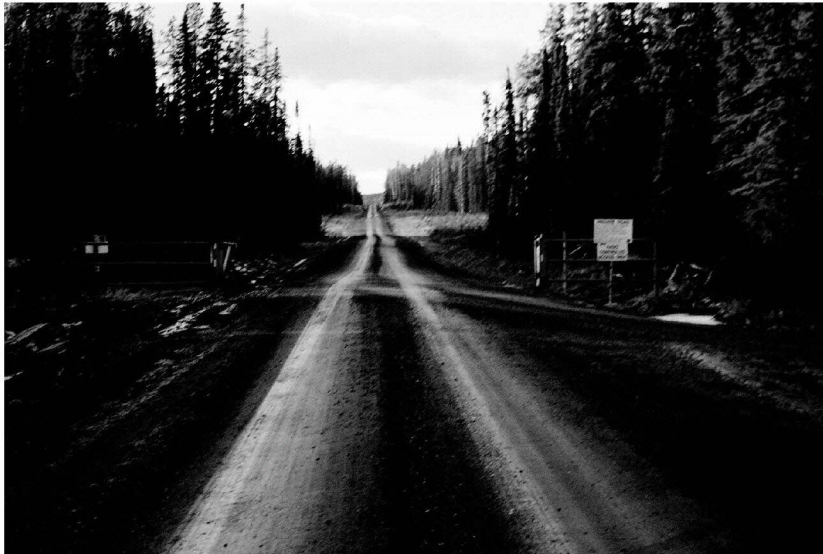
Photo No. 1: Entrance to Mainline Road off Route 752 (5 November 2002)
