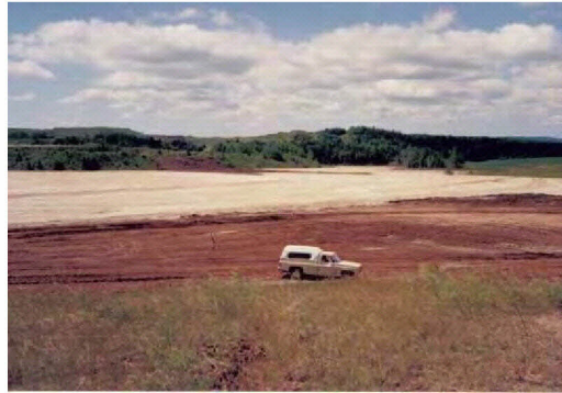
Photo 5.6-8: Topsoil placement - Early 1990s
