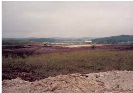
Photo 5.6-9: Topsoil placement - Early 1990s
