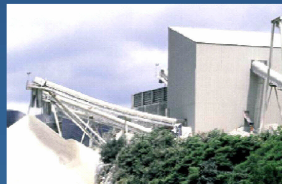
Example: enclosed crushing structure
