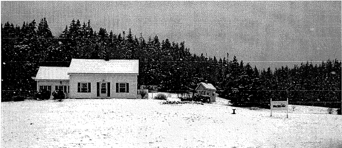
Bilcon's office at the Towle House in Little River
