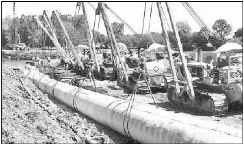
Figure 9. A wet crossing
