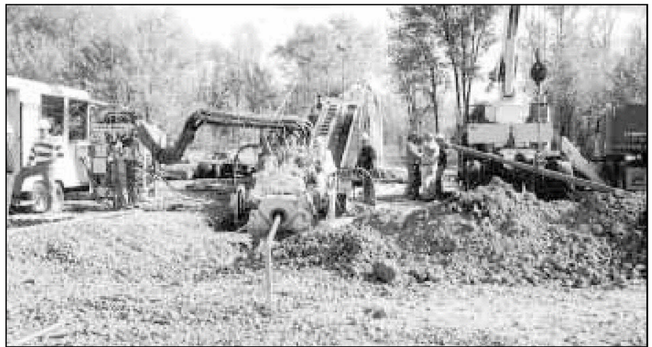
Figure 10. A directional drilled crossing
