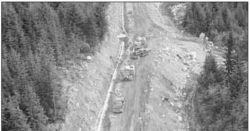
Figure 14. Photograph of Pipeline Construction Activity
