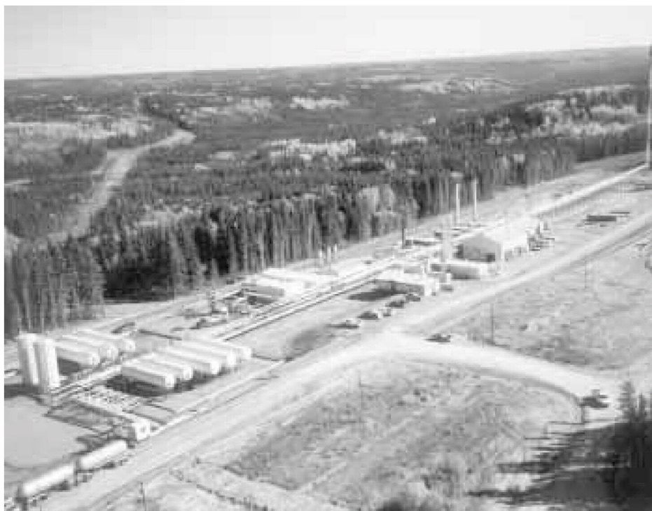
Figure 5. Photograph of a Typical Gas Plant
