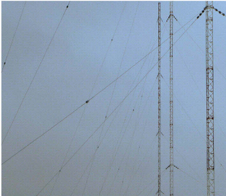
Guy wires increase the volume of sky a tower intercepts. Photo © Martin Damus
