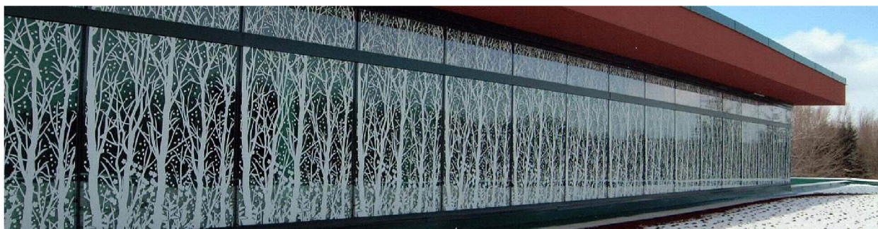
Another view of the windows with the applied cut film. Photo © FLAP.
