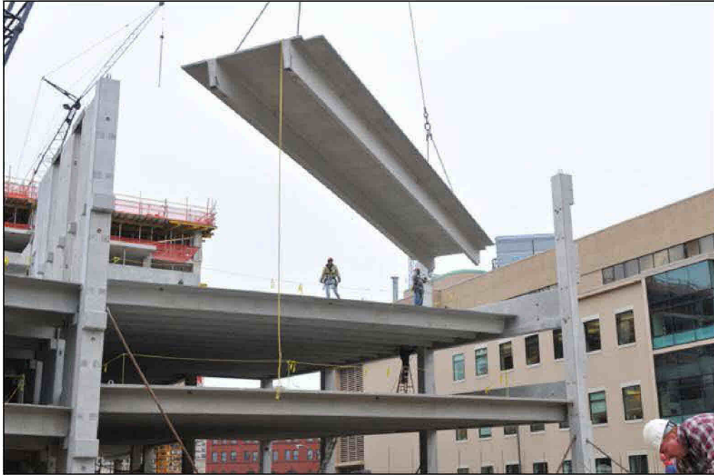
Pre- cast “double T” deck for parking garage
