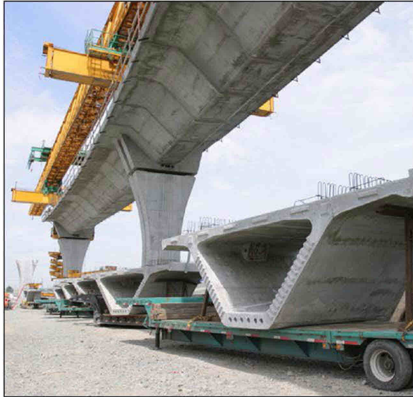
Pre- cast bridge deck sections
