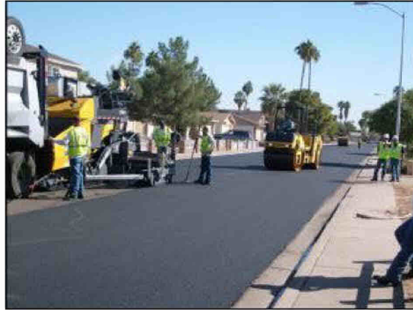
Paving Machine with Roller in Background
