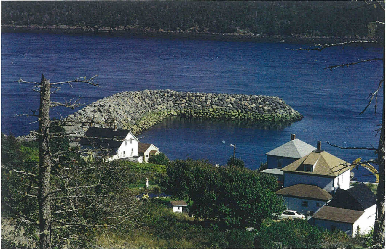
Figure 9. A recently constructed breakwater made from basalt armourstone at Tiverton, Digby County.
