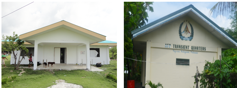
These comprise one (1) Municipal Health Center capable to house five (5) patients at a time and a Transient House for guest of the Armed Forces of the Philippines.
