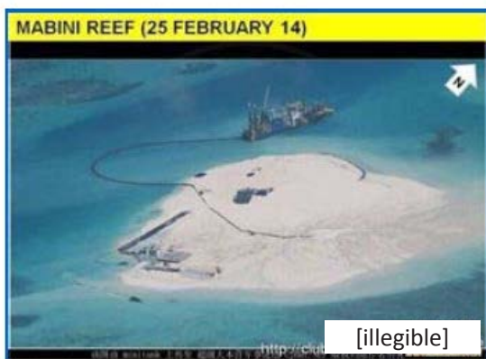
Tianjing’s worksite at Chigua Jiao
