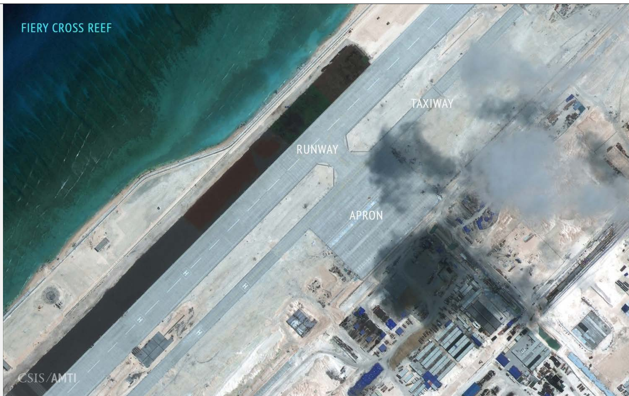
FIERY CROSS REEF. September 3, 2015. Runway completion and painting at Fierly Cross Reef. A large apron and taxiway is clearly visible.
