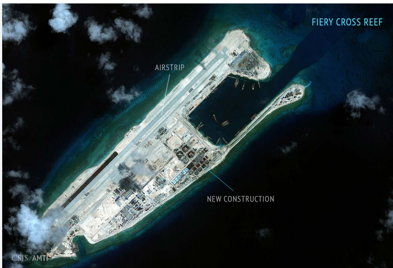
FIERY CROSS REEF. September 3, 2015. Runway construction nears completion as paint is applied to the concrete on the western side of the reef. New building construction has appeared on the east side of the reef.
