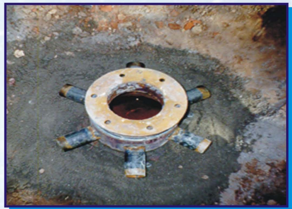
A T used to join the well points with the pump
