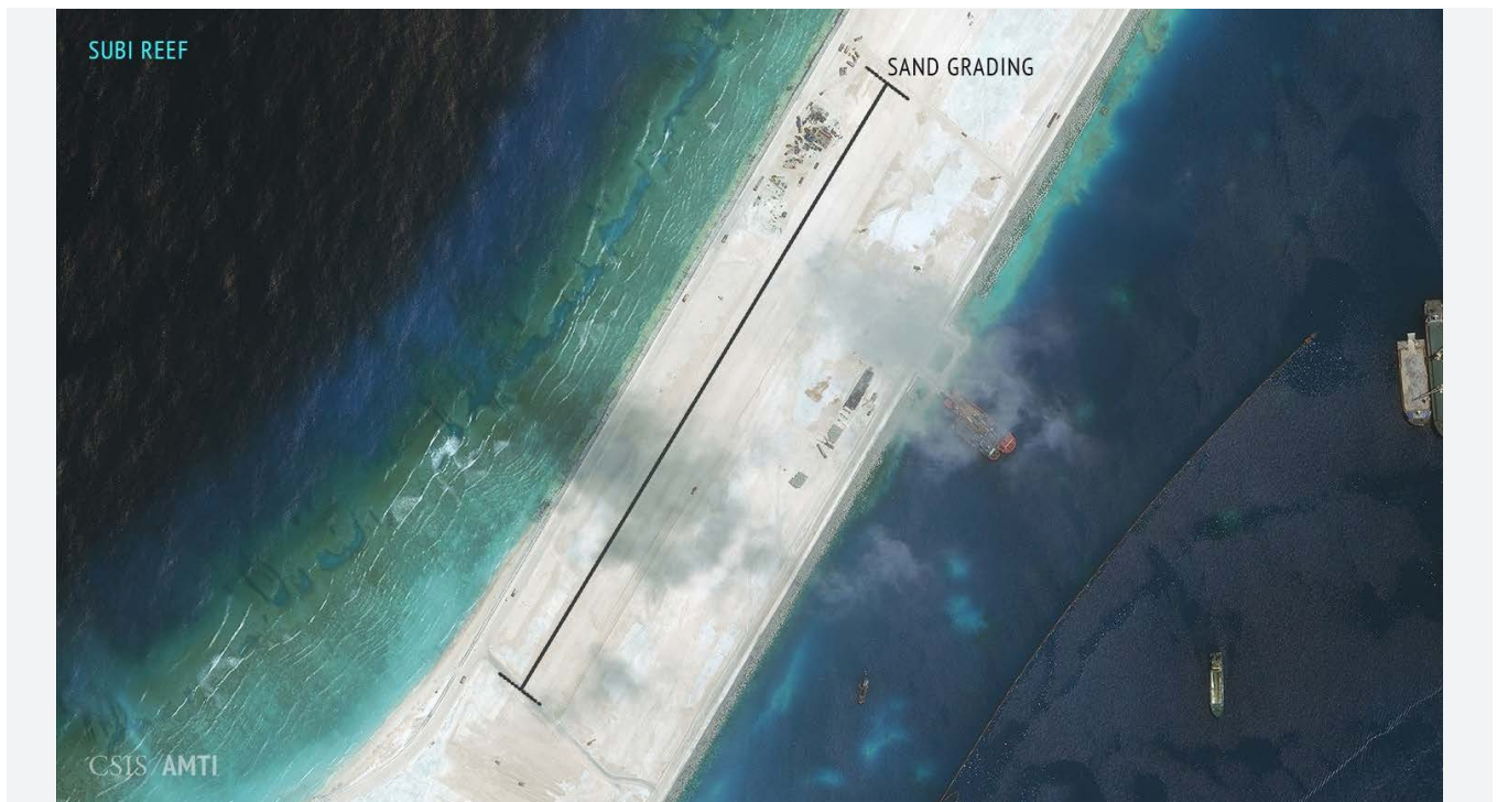
SUBI REEF. September 3, 2015. Possible airstrip construction at Subi Reef.
