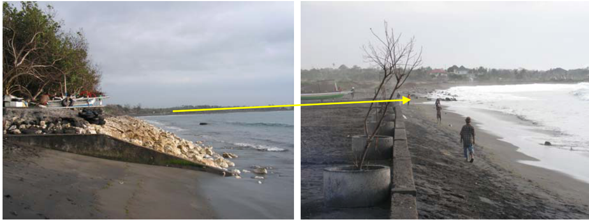
Plate 4.2 Coastal protection efforts to protect a valuable tourism base; meanwhile, the adjacent shore with less economic value has minimal and improper protection. Even revegetation with waru to replicate planting at the neighbouring resort failed; the coast was then abandoned and left to erode
