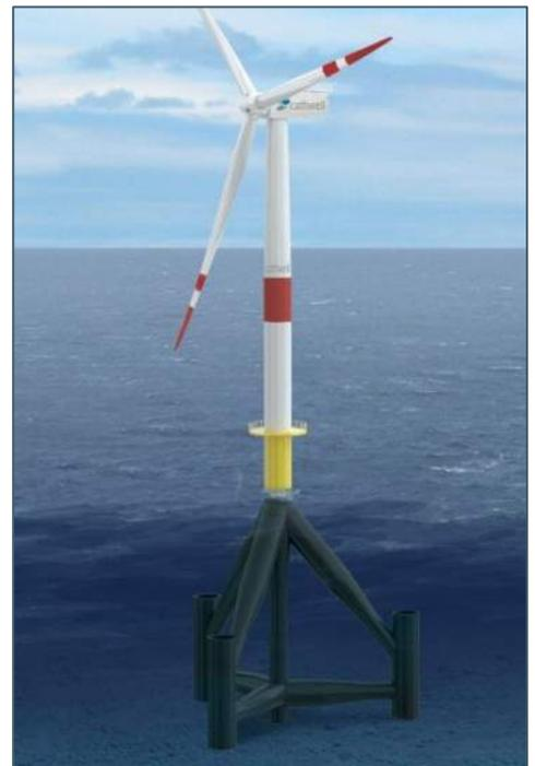
Figure 4-10 (Right): Tripod foundation rendering (Courtesy of Cathwell)
