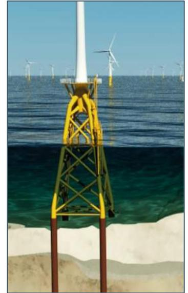
Figure 4-5 (Left): Wikinger OWF jacket foundations, Nov. 2016 (Courtesy of Bladt)
