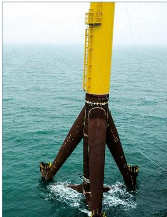
Figure 4-9 (Left): Global Tech 1 OWF tripod foundation (Courtesy of Global Tech 1)
