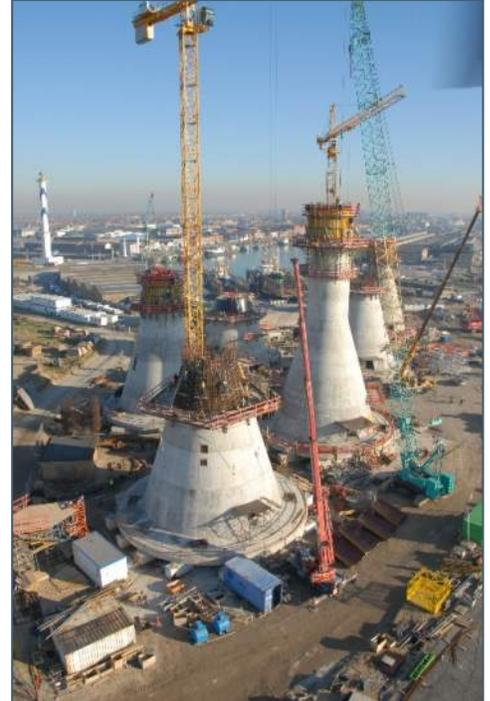
Figure 3-4 (Right) Thornton Bank Offshore Wind Farm GBFs under construction, Feb. 2008
