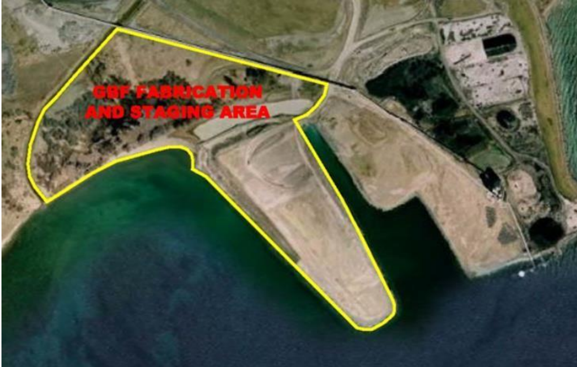
Figure G-9: St Mary's Cement Facility Bowmanville, Ontario
