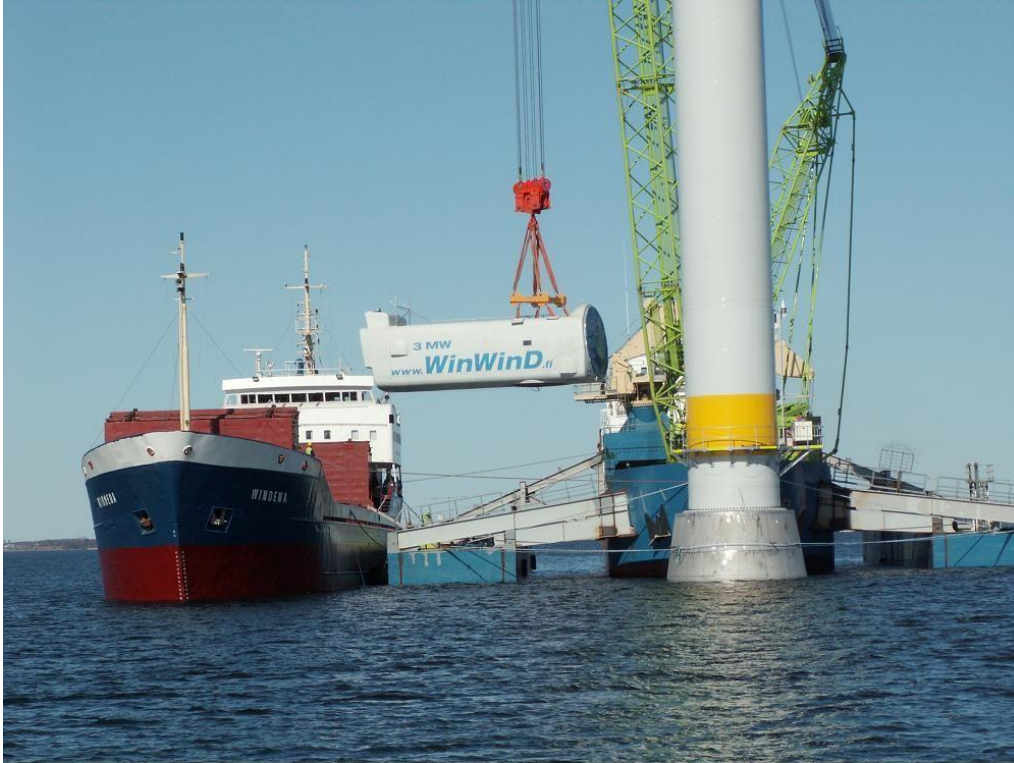
Figure 2-6: Lake Vänern Wind Turbines Installation
