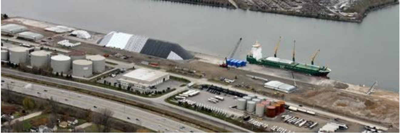
Figure J-33: Pier 26 Hamilton Ontario
