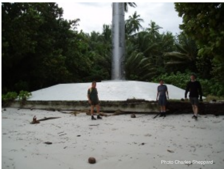
Eastern Diego Garcia, lagoon shore, where a large navigation marker now abuts the beach with undercutting of its foundation.
